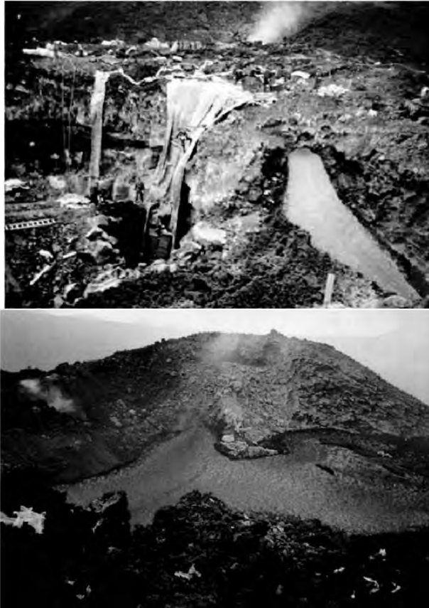
Figure 1. The control of lava flows. Significant progress achieved at Mt. Etna in the last 20 years. Left: Diversion of the flow into an artificial channel by blasting its levee near the eruptive vent. Right: Deprived of back-thrust, the natural flow front stops. A new flow originates from the diversion site
