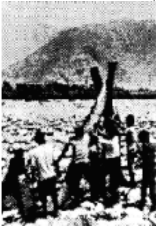
Community-based mitigation strategies tend to maximize the use of local resources; materials, labor and management.
